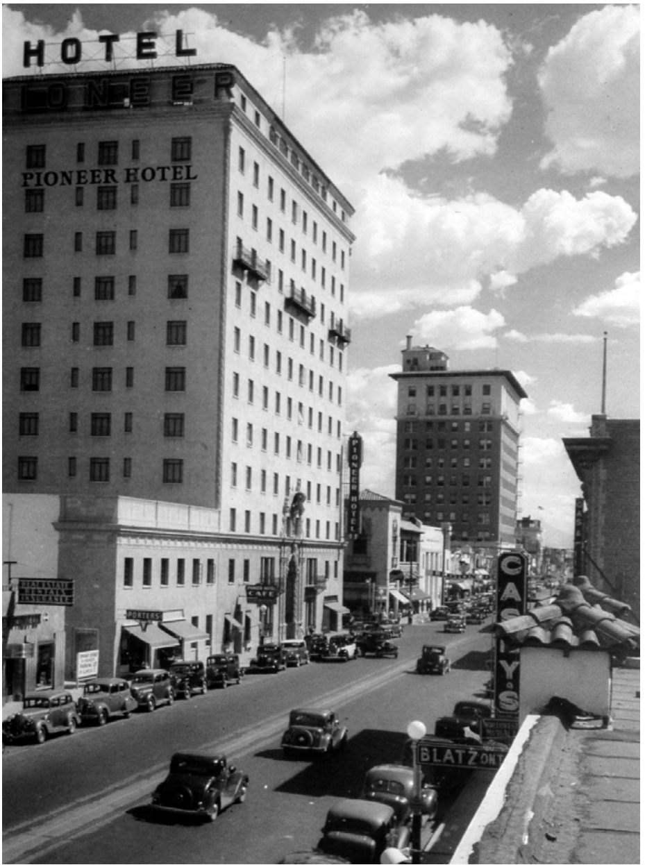
Stone Avenue, Tucson, in the 1930s. Arizona Historical Society
